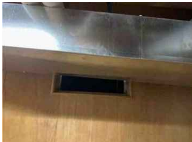
Crawl Space Access
