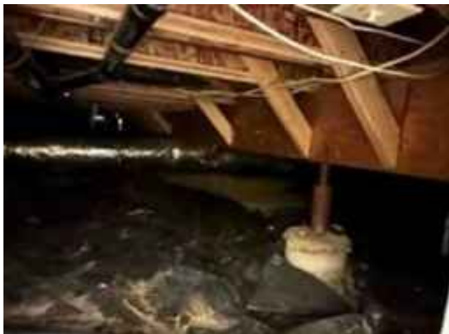
Attic Crawl Space
